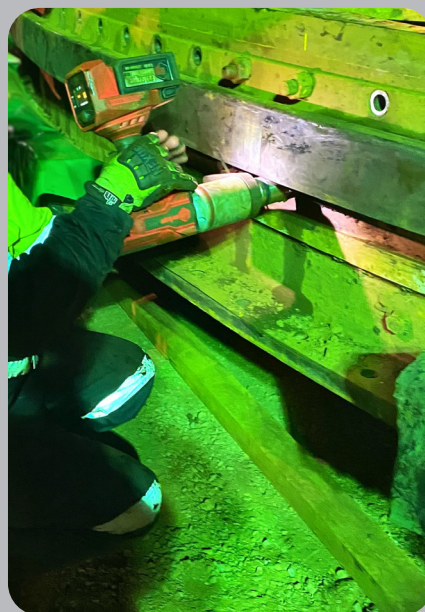
Rotary O-section bolt installation
